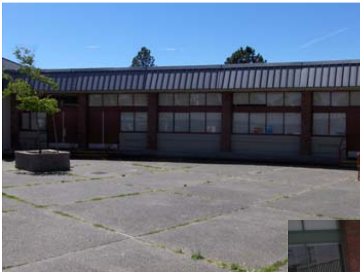
The courtyard, Spring 2007, pre construction
